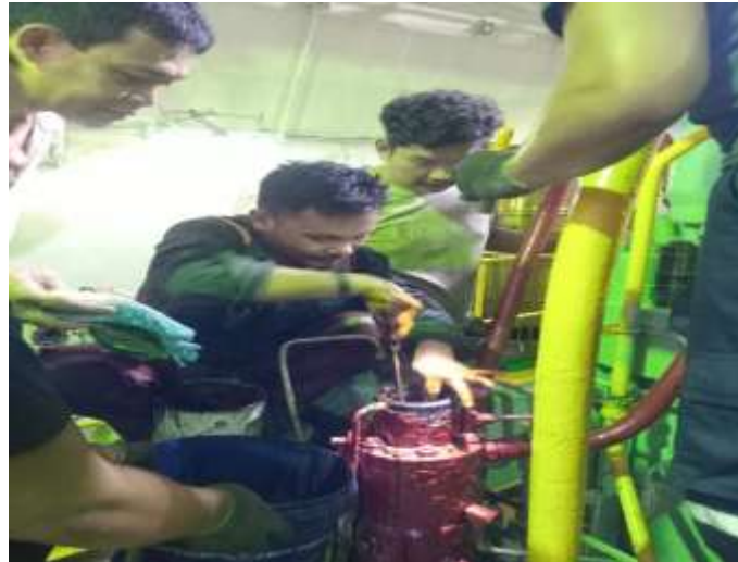
Fig. 5. the process of replacing a problematic puncture valve
