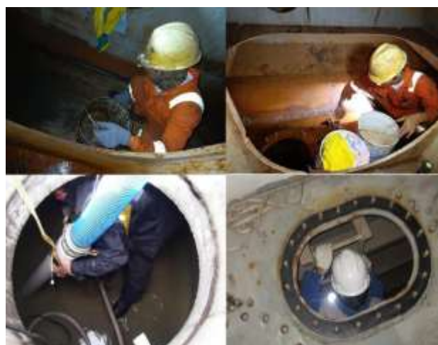
Picture 8. Maintenance Ballast Tank
