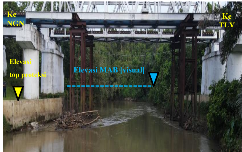
Figure 6. Position of MAB on the bridge structure
